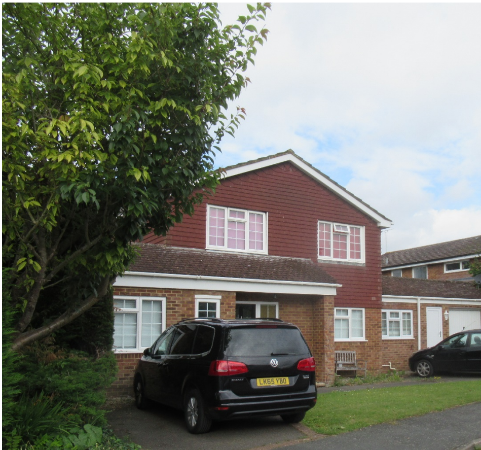
Front elevation of 8 Orchard Close
